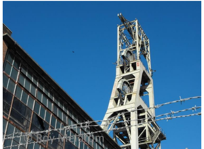
Clipstone No1 Shaft Headstocks (March 2010)
