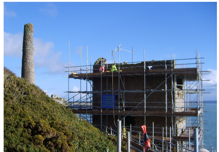
Conservation work underway at Trewavas Mine in Cornwall - photo: Kevin Baker
